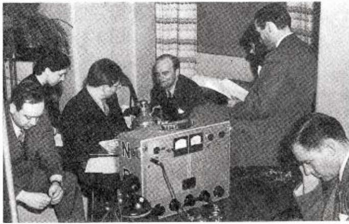
WHEN Edgar Bergen was confined to St. Vincent's hospital, Los Angeles, Dec. 10 with an infected face, NBC Hollywood engineers proved that when the show must go on against unexpected odds, it can still be done the easy way. Lines were quickly put into the hospital room and Bergen with Charlie McCarthy were very much a part of the NBC-Red Chase & Sanborn Hour. Left to right are James Bealle, publicity director of J. Walter Thompson Co., agency servicing the Standard Brands account; Mary Hanrahan, secretary to Mr. Bergen; Dick Mack; Mr. Bergen; Joe Parker, NBC director, and Paul Green, NBC technician.
